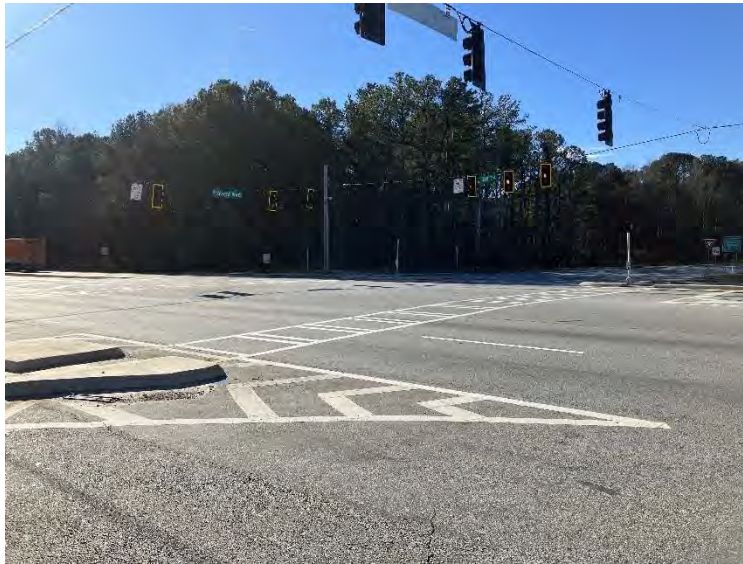
The south corner of Fairburn Industrial Boulevard and Howell Avenue
